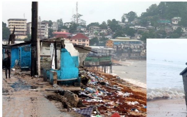
Coastal erosion at West Point Township has destroyed recently built sanitation facilities
